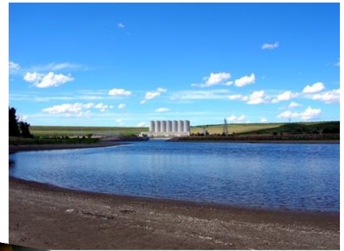
Oahe Dam Power Plant
